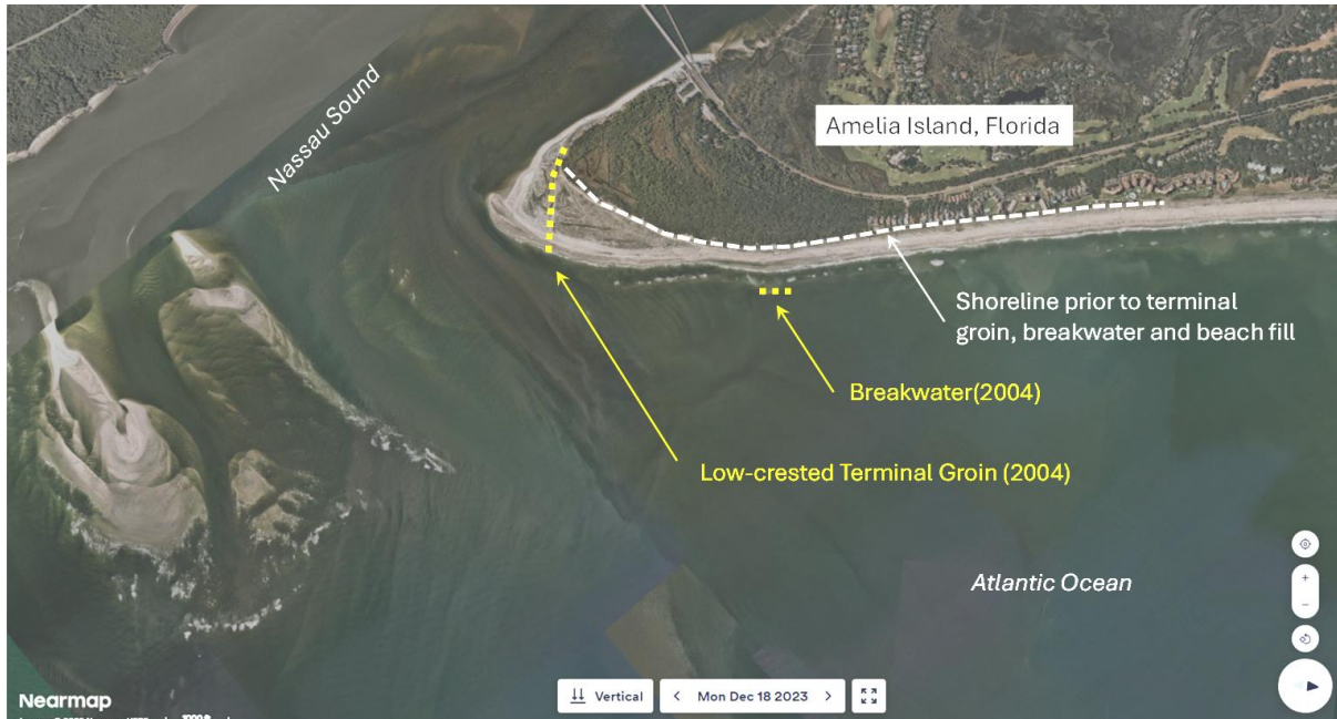
Figure 15: Example at the southern end of Amelia Island, Florida of a low-crested terminal groin and updrift detached breakwater to address chronic shoreline erosion that could not be addressed with beach nourishment alone due to excessively high erosion rates. This project has reduced sand loss rates along the southernmost end of Amelia Island to a level that allows typical beach restoration along the southern end of the island to be a successful beach management application.
