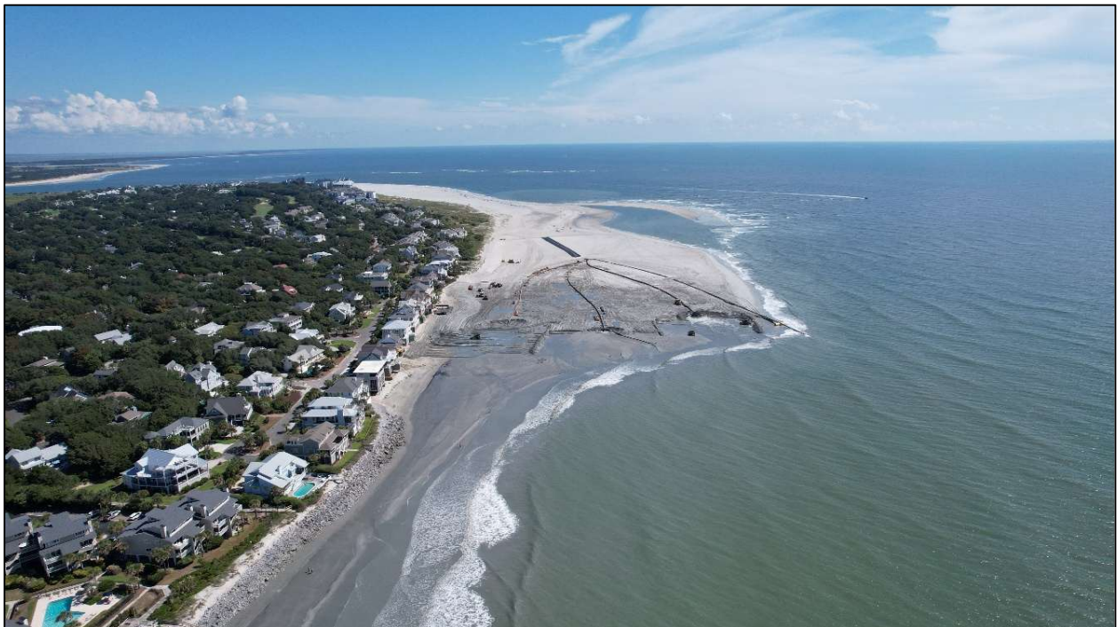
FIGURE 1. Reach 1 was completed on 30 August 2026 and mobilized to Reach 2 shortly after. At the time of writing this report Marinex is working in front of Grand Pavilion ( image collected 21 September 2026 ).
