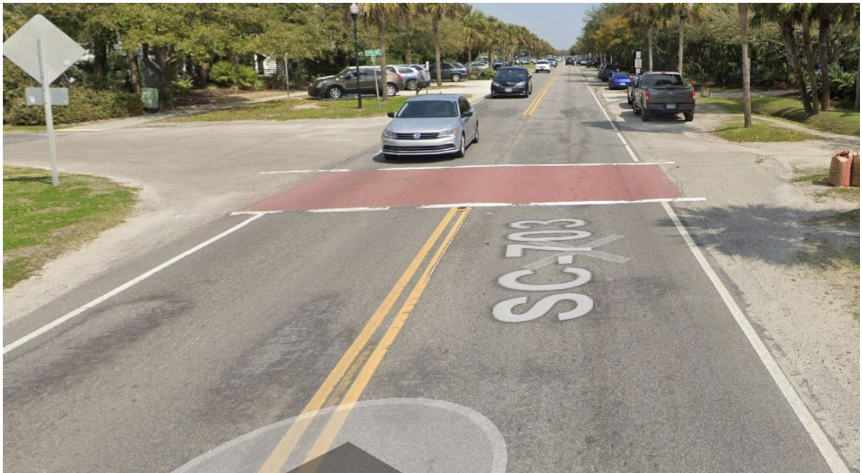
Figure 8. 25 th Avenue. Does not appear to meet preliminary SCDOT site criteria.
