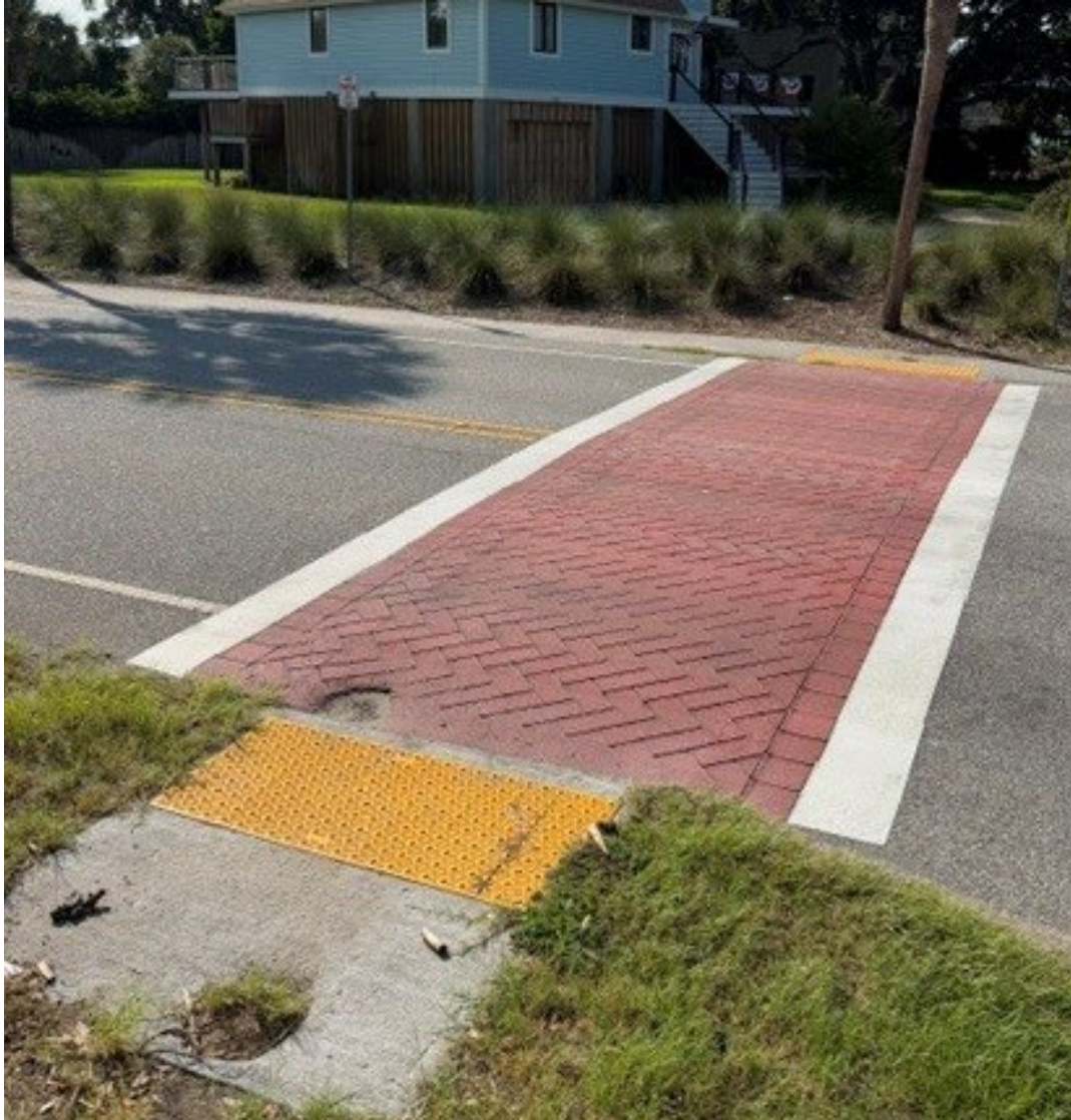
Figure 13. 43 rd Avenue. Appears to meet most preliminary SCDOT site criteria.
