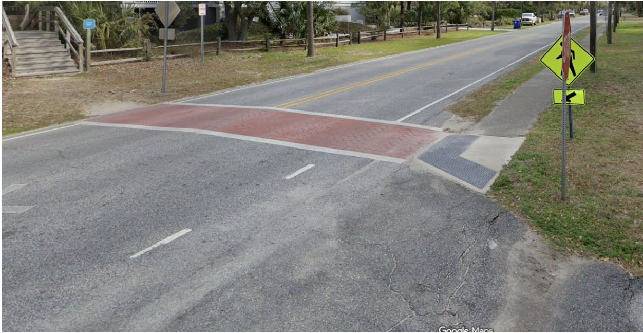
Figure 15. 49 th Avenue. Appears to require substantial improvements to meet preliminary SCDOT site criteria.
