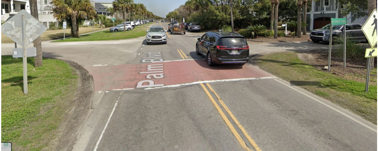
Figure 11. 34 th Avenue. Does not appear to meet preliminary SCDOT site criteria.
