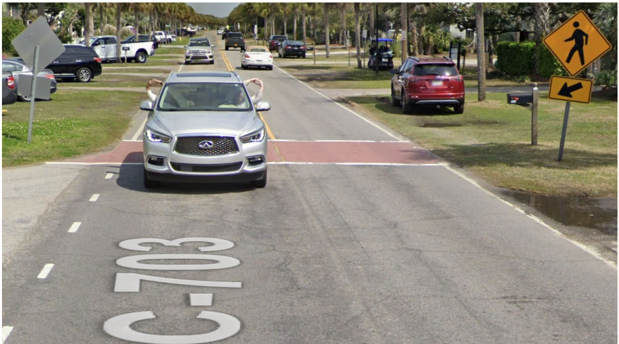
Figure 10. 31 st Avenue. Does not appear to meet preliminary SCDOT site criteria.
