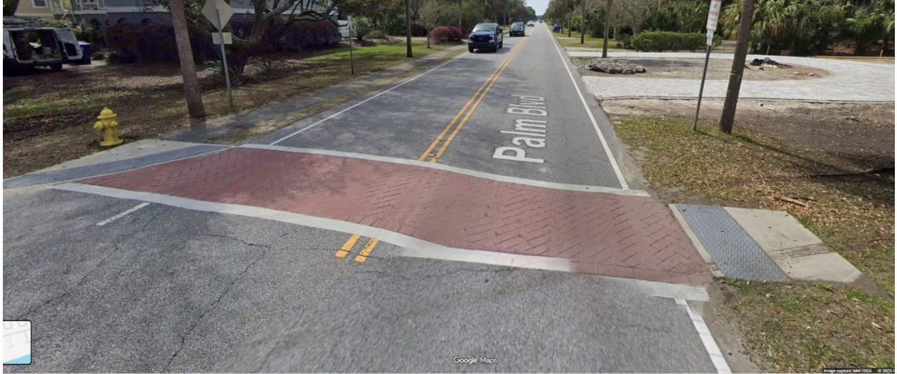
Figure 17. 53 rd Avenue. Appears to meet most preliminary SCDOT site criteria..
