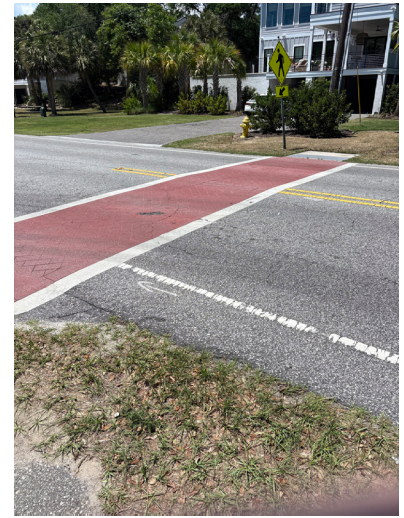
DELINEATED CROSSWALK WITH PEDESTRIAN CROSSING SIGN
