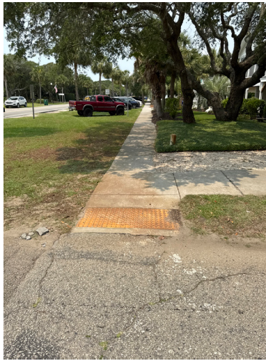
AT-GRADE SIDEWALK WITH TRUNCATED DOMES
