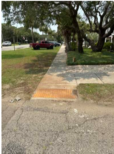
AT-GRADE SIDEWALK WITH TRUNCATED DOMES
