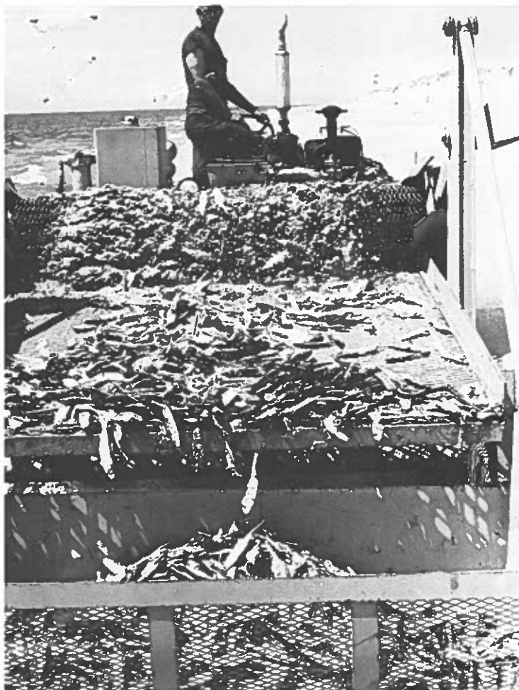
Separating the shad from the sand. A BeachLeach rids a section of Lake Michigan shore of the alewife problem during 1967 "invasion."
