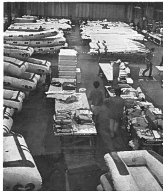
View down length of shop shows stacked slides.
